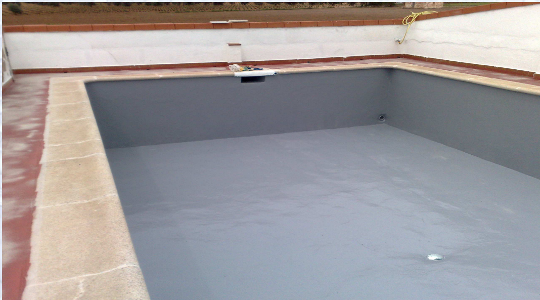
During application process
